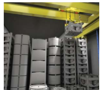
NDA image of a vault in a repository for intermediate level waste
