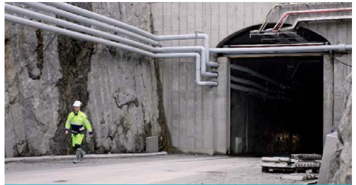
Entrance to a repository being built in Finland (Posiva)
