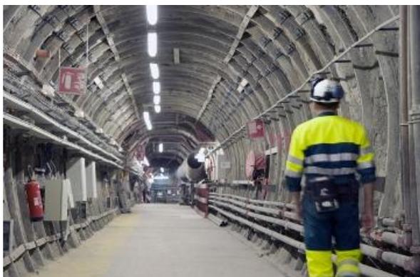
The laboratory has been built to test the suitability of the area for a possible geological disposal facility for higher activity radioactive waste.
