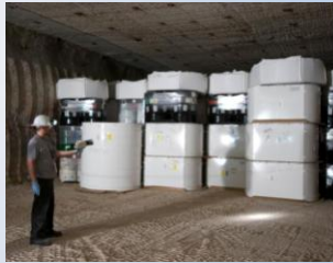
CH waste is disposed in columns on the disposal room floor. Disposal began in March 1999.
