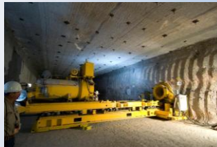
RH waste is disposed in pre-drilled boreholes in the walls of the disposal room and sealed with a concrete shield plug. Disposal began in January 2007.
